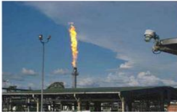
FLARE (before OGE&EE Project)
